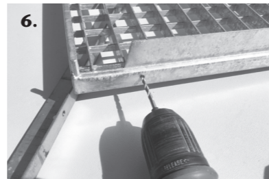
6. Pre-drill using a 4 mm drill
