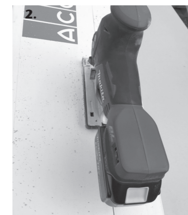
Use a jig saw to cut the extension element to length. Remove reinforcement bars if necessary first.
