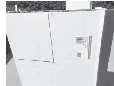
1. Remove the wall connection profiles and mark the notch
