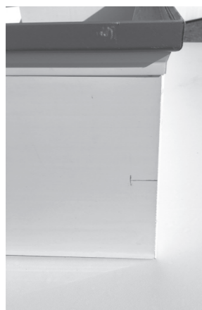
Determine the position of the reinforcement bars and mark the profile thickness (35 mm).
