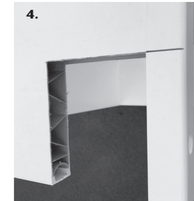
4. Slide the wall connection profile in place and cut to size
