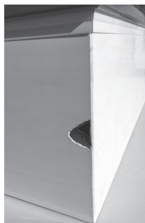
Open the section chambers using further drillholes so that the reinforcement bar can be removed.
