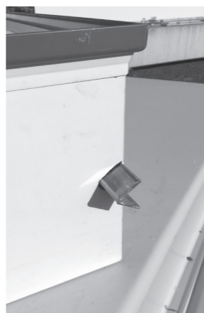
Remove reinforcement bar
