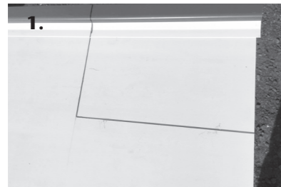
1. Remove wall connection profiles. Mark the area to be notched
