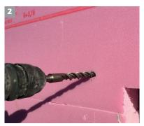
If the drilling installation aid is not on hand, hold the light shaft with the grating inserted against the wall and mark the two upper fixing points. To remain flexible in the height position, the two upper fixing points can also be set somewhat lower within the rectangular hole. Now drill the holes using a 16 mm drill.
