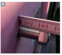
Drive the heavy-duty anchors with nut screwed in place into the wall or through the insulation into the wall. The heavy-duty anchor should protrude by approx. 4.5 cm.
