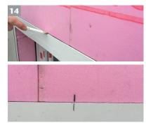
Mark the horizontal rear wall position on the insulation or wall. Mark the vertical rear wall position on insulation or wall and rear wall. Remove the rear wall and the light shaft.
