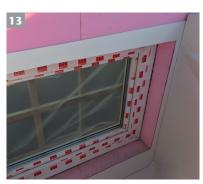
Remove the rear wall. Cut the window recess out using a jig saw. Remove the protective film. Slide the rear wall back in again and align it.
