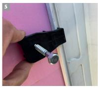
Hold the guide block in place between the two marks (arrows). Mark the fixing point using a screw.
