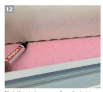
Mark the window recess from the inside. Use the insulation for guidance. Take the outside dimension of the insulation connection profile into account. Cut the insulation if necessary.
