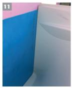
Slide the rear wall in the light shaft groove on the wall side.
