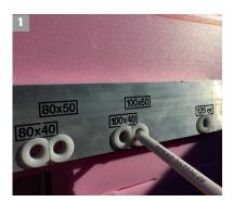
Mark the top edge of the light shaft in relation to the top edge of the ground. When the ACO drilling installation aid is used, top edge drilling installation aid = top edge light shaft. The distance between the bottom edge of the window to the light shaft base should be at least 15 cm. Mark the two upper fixing points.
