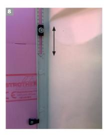
The locking block is moved to the slide position by lifting and turning through 90 degrees. Now the complete light shaft body can be moved up or down.
