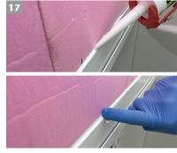
Apply sealant again in the transition area from rear wall to insulation or wall. Smooth the sealant.
