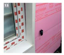
Assemble the insulation connection profile according to the assembly instructions. Remove the frame seal. Slide the insulation connection profile through the rear wall and insert it in the frame groove.
