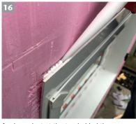
Apply sealant at the top behind the rear wall. Align the rear wall according to the markings and press in place. Screw the light shaft in place. Check the position of the rear wall again. Correct if necessary.
