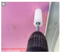
Screw the spiral anchor in flush using the screw head. When installation is directly on the wall, drill a 10 mm drillhole and drive the anchor in. If the insulation is less than 10 cm thick, screw the anchor in slightly and then remove it again. Shorten the spiral anchor according to the insulation thickness and screw it in flush.
